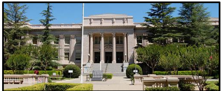
Marina Courthouse - electrical updating $36,800
